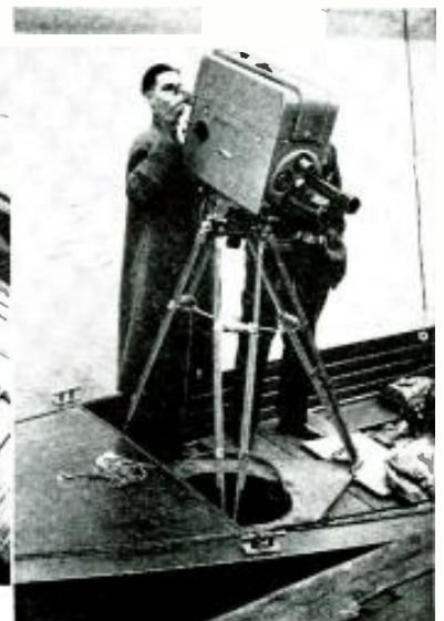
The television-transmitting launch Consuta . Camera control equipment on the launch. Marconi camera on its vibration-free mount.
